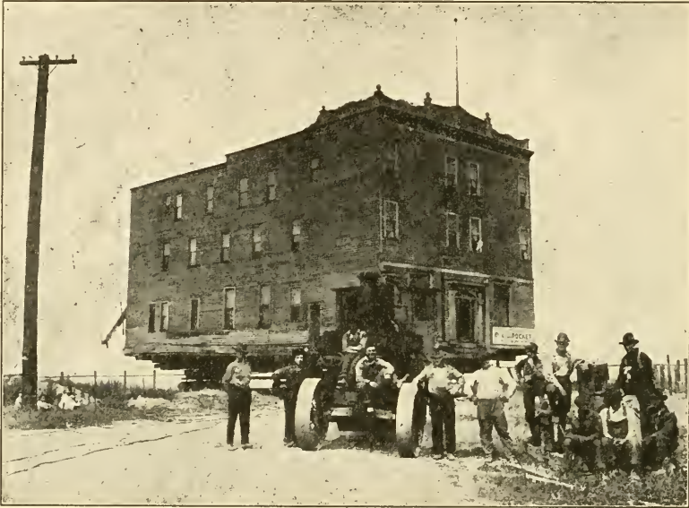
A CONCRETE-FLOORED BUILDING MOVED SUCCESSFULLY TO NEW HIBBING—THE OLD COLONIA HOUSE, ON ITS WAY TO NEW SITE, THERE TO BE RENOVATED AND RENTED TO SCHOOL BOARD AT $500 A MONTH, FOR USE AS TEACHERS' APARTMENT HOUSE
